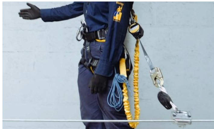
Correct setup of fall protection devices when working on container roof
