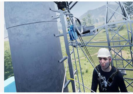
To perform this exercise, you will need a harness, a descent device, a work positioning lanyard, some tape slings, and a double fall arrest lanyard.
