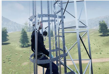
To perform this exercise, you will need: a fall arrester, a descent device, 2 ropes of 30 m, some tape slings, and a work positioning lanyard.
