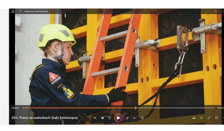
VRAPP at Height makes it possible to practice using safety hooks suited to the particular formwork type.
