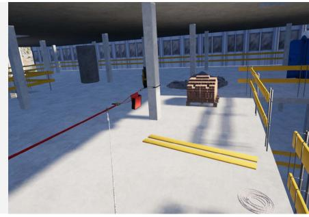
To perform this exercise, you will need a harness, the horizontal safety system, and a rope with a fall arrester.
