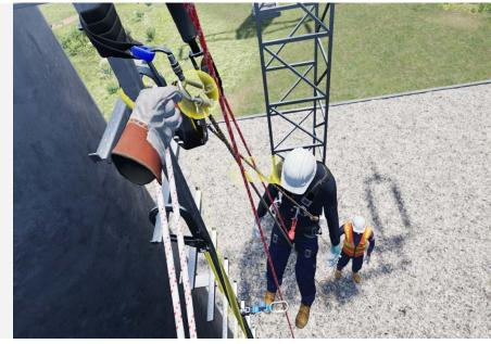
To perform this exercise, you will need: a fall arrester, a descent device, 2 ropes of 30 m, tape slings, and a work positioning lanyard.
