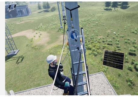
To perform this exercise, you will need: a descent device, a work positioning lanyard, some rope and a fall arrester, some tape slings.
